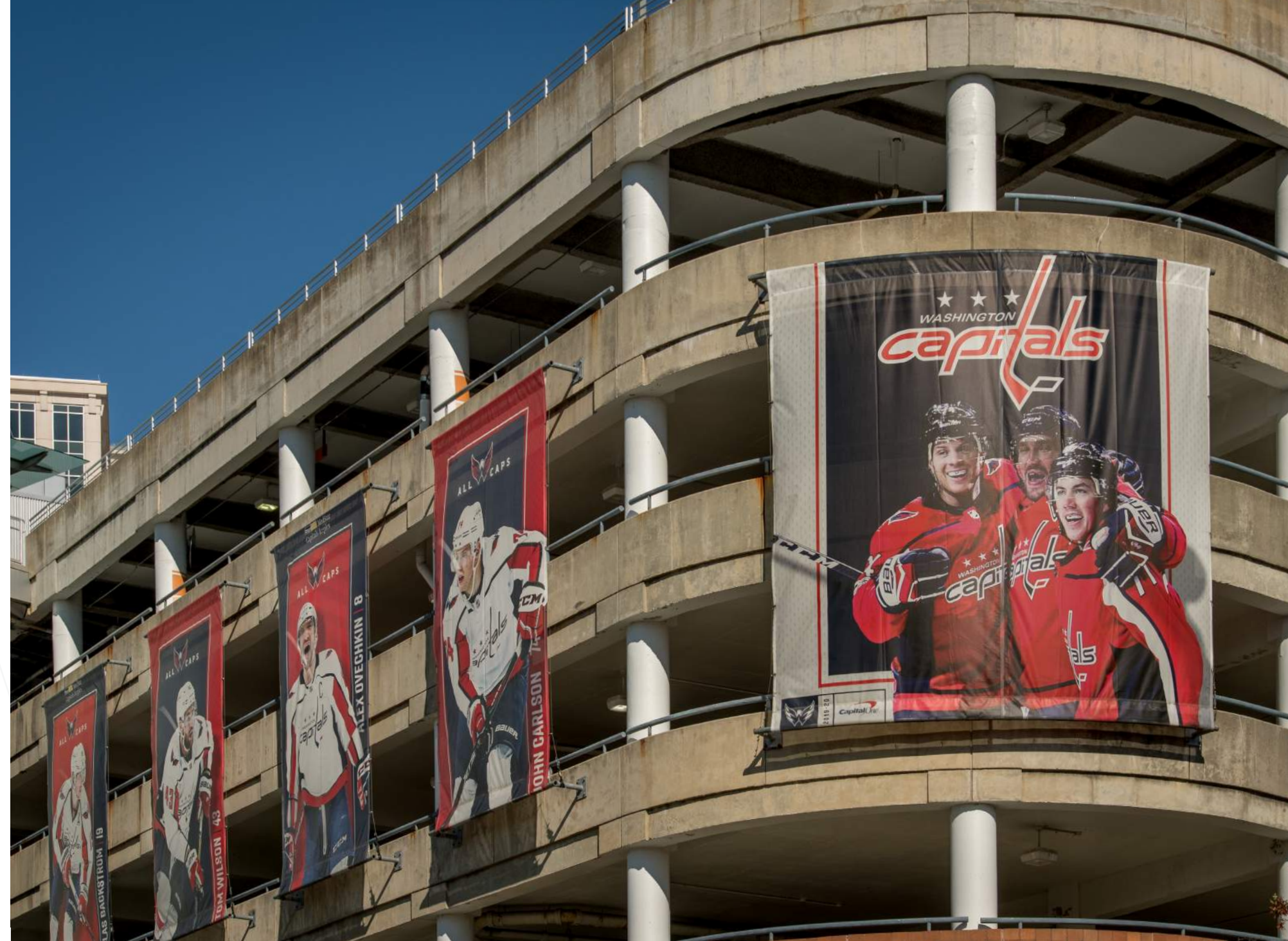
EXISTING BANNERS ON ICEPLEX PARKING GARAGE
